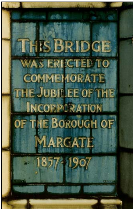
Close-up of one of the panels on the 'new' bridge
