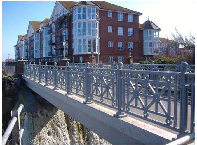
A general view of Newgate Gap Bridge showing the ornamental ironwork
